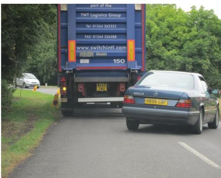
At the point where lorries are now required to stop, the edge of the tarmac has broken down, as has the grass verge and mud has been spread on the carriageway, which is both unsightly and unsafe. In addition an existing road sign is obscured by the parked lorries.
